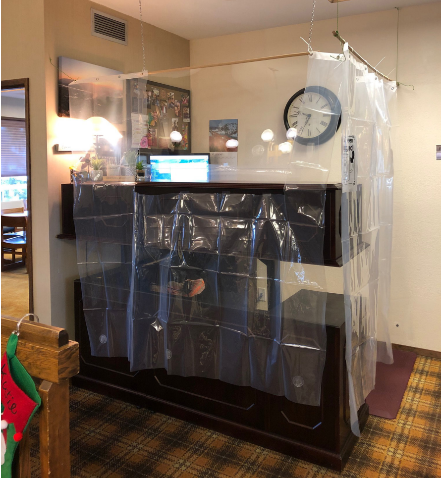
An example of the protective barriers installed at the district office. Initially, building staff began using plexiglass barriers, but due to their high cost and limited availability, the district switched to using clear plastic shower curtains.
